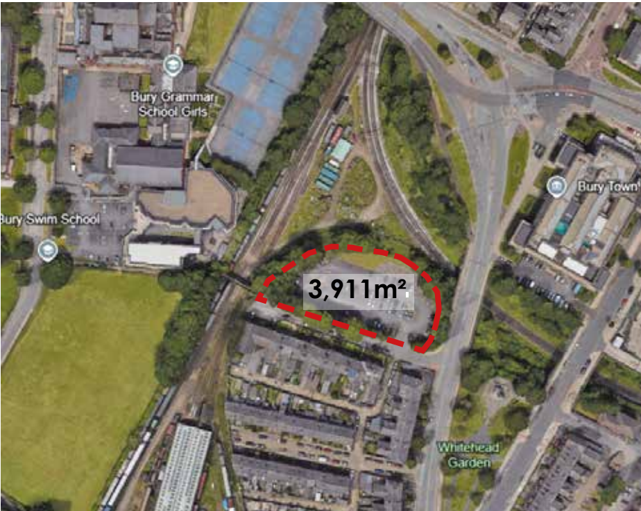
Figure 1.1 Existing Site (Google Map), Date: 2024.11.06)
